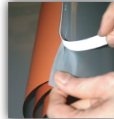
6. REMOVE PVC STRIP, LEAVE LOOP TAPE ATTACHED.
